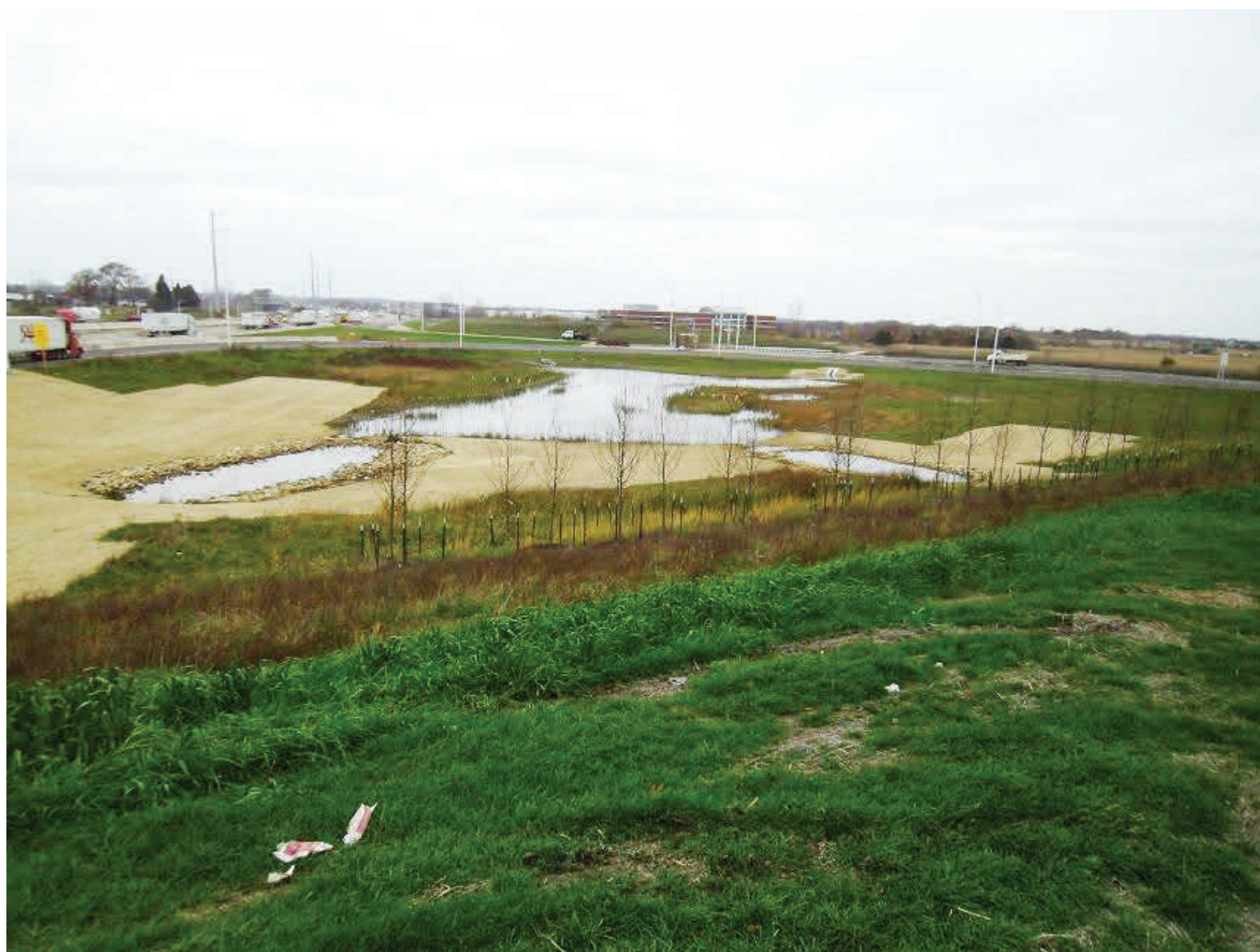
Illinois Route 47 Interchange on the Jane Addams Memorial Tollway (I-90) bioswales and stormwater detention areas.
